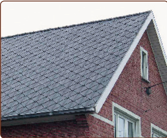
Dakleien in asbestcement
